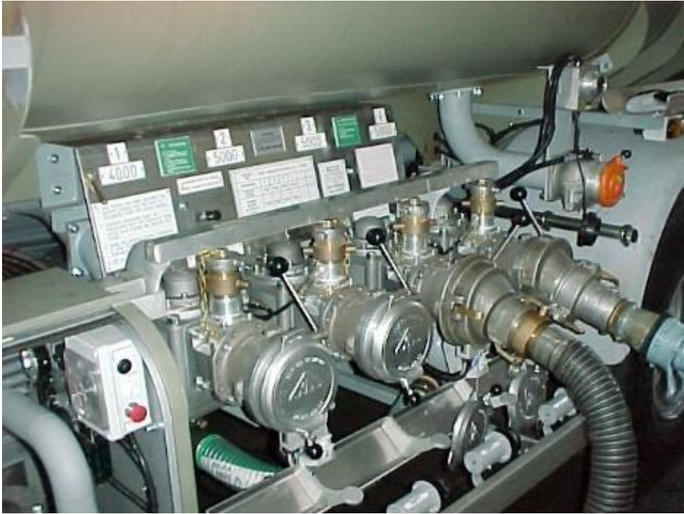
Underside of Manifold
